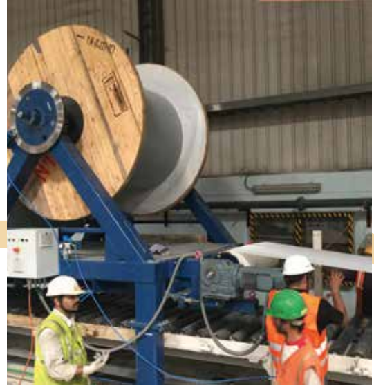
Wednesday, 5 p.m. Now it's time to really get going. The new PVC belt is on the special winding device provided by us and is inserted into the conveyor.
