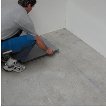
The installation of Colorex Plus starts with the second row of tiles from the wall.
