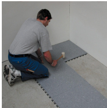
A rubber mallet can be used for engaging the connection system.
