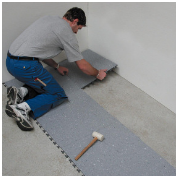
Once the second row is complete, the first row is measured and fitted.
