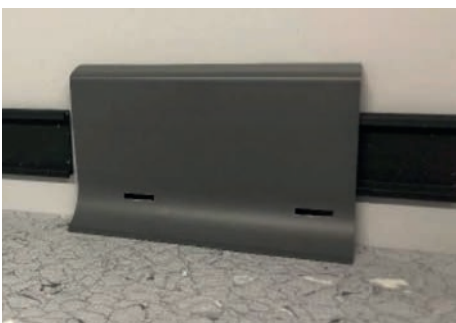
Ventilation part: Colorex Plus must be cut 5mm before the wall
