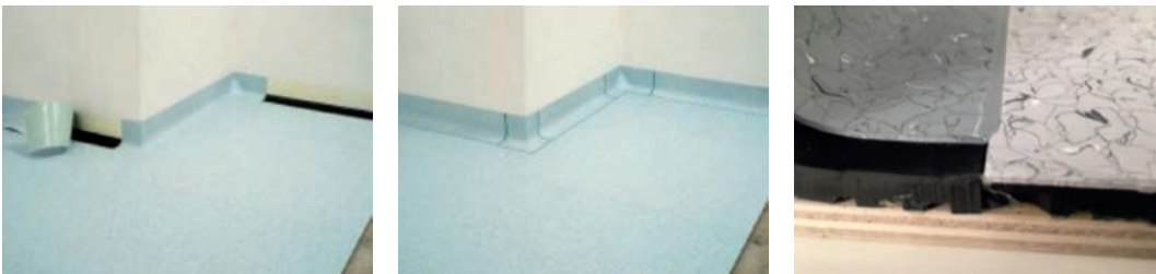
Welded cove former and tile
