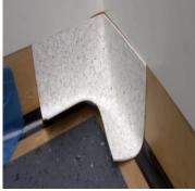
Try to keep the piece from the floor. At this point remove the protection and apply the other side while keeping the lower side from the floor.
