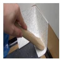
Press well, heat the lower part and press it down to the floor.
