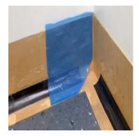
We suggest to cover one side to avoid that the glue interferes with the correct application of the corner
