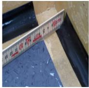
Install the floor leaving 5 cm distance from the wall
