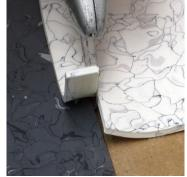
The lower part will overlap the floor by about 1cm. this will allow to cut it properly to be aligned with the floor. This will allow to cut it properly to be aligned with the floor.
