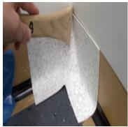
At this point remove the protection and apply the other side while keeping the lower side from the floor.
