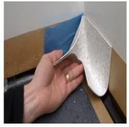
After having well heated the piece with a hot air gun, position the side respecting the height sign [10 cm].
