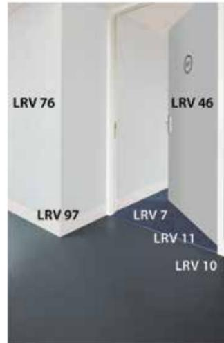
It is not always possible to achieve 30 degrees of contrast between walls, skirting and floors. When this is the case, it is essential that optimum contrast is achieved between the two critical planes; the floor and wall.
