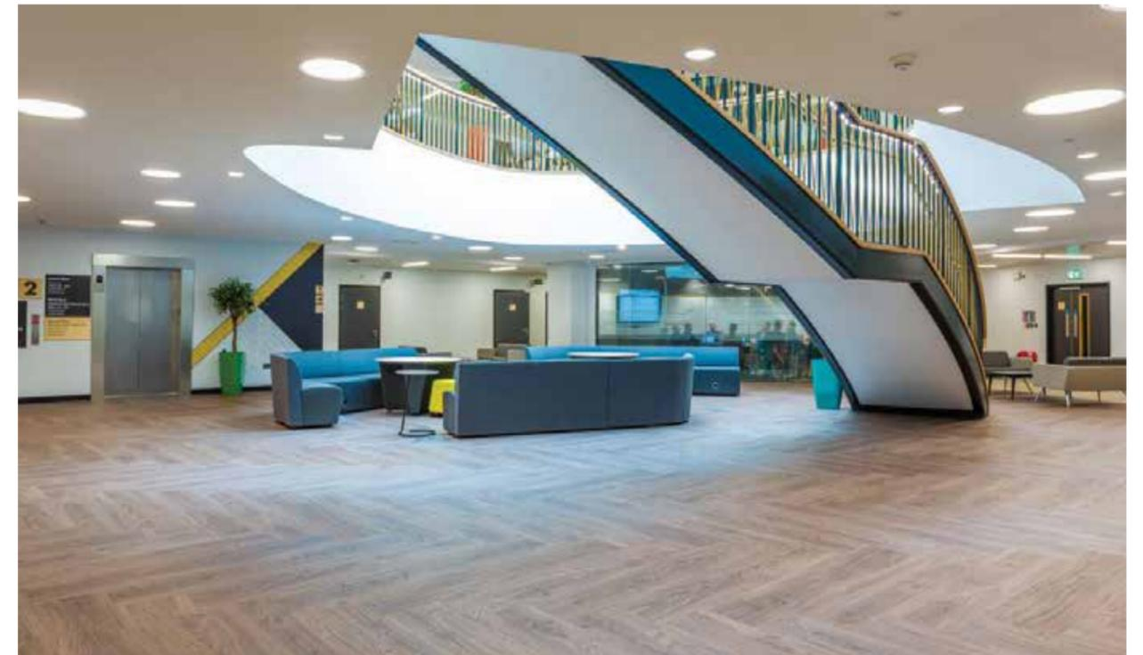
Allura Wood LVT in the Vintage Oak colourway was used for the staircase, main circulation areas and breakout spaces on each floor; achieving one tonally continuous flooring surface. In addition, our Surestep safety vinyl in Beton Concrete was used in areas where there is an increased slip risk, such as the toilets, kitchens and tea points.
