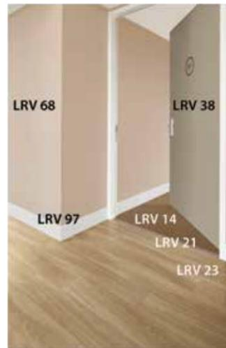
Adjoining flooring should not contrast more than 10 degrees of light reflectance value. In this example there are 9 degrees of contrast between the two floors.
