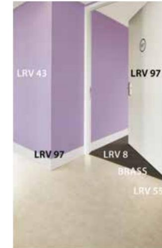
Highly reflective trims create glare. The ageing eye is more sensitive to glare and often, the glare from the strip can be perceived as a step, resulting in high-stepping. For some people with dementia, the highly reflective strip can deter the person from passing.
