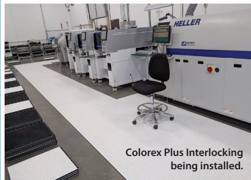
Colorex Plus Interlocking installed over access panels.
