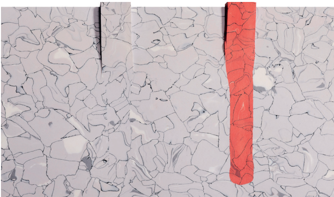
A piece of Colorex can be used for a seamless repair
