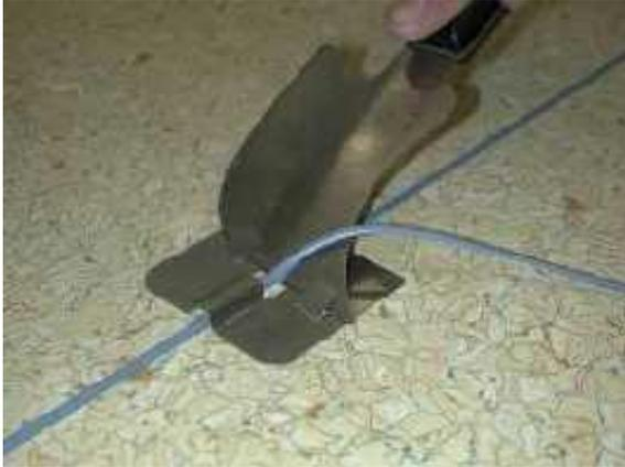
4. The welding cable will dish slightly (concave downwards) as it cools. Wait until the material is completely cool before carrying out the final trim, trimming flush with the surface of the sheet with a sharp spatula angled slightly across the line of cut or a Mozart knife (with the spacer plate moved to one side).
