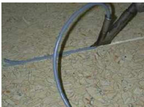
3. The first trim of the weld cable should be carried out while the cable is still warm.
