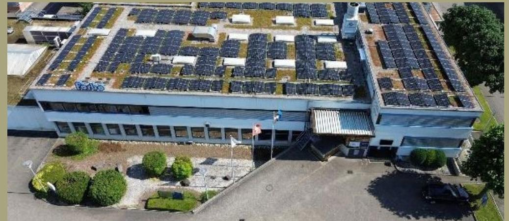
Some 391 very efficient photovoltaic modules were installed on the roof of our production shed at the Wallbach site.
