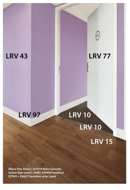
Where it is possible to abut flooring without a transitional strip, this is preferred, as this will reduce the number of interfaces to be coordinated. However, ensure the flooring is level; floor thicknessses can vary.
