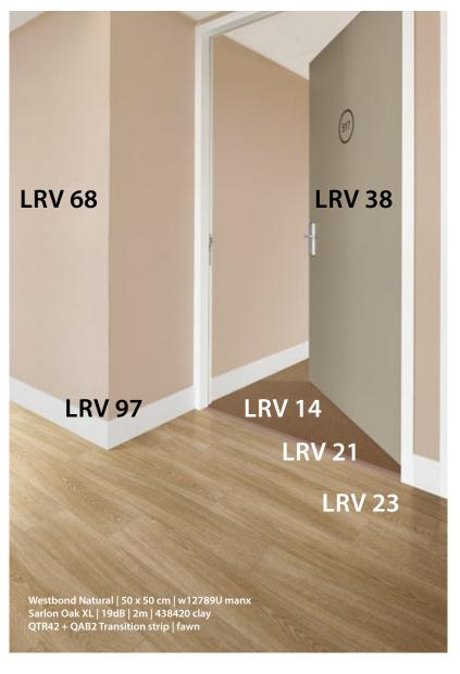
Adjoining flooring should not contrast more than 10 degrees of light reflectance value. In this example there are 9 degrees of contrast between the two floors.
