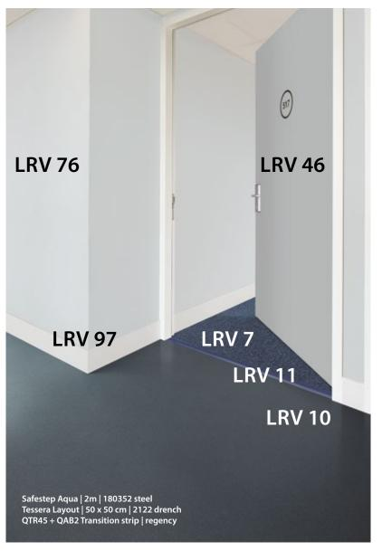
It is not always possible to achieve 30 degrees of contrast between walls, skirting and floors. When this is the case, it is essential that optimum contrast is achieved between the two critical planes; the floor and wall.
