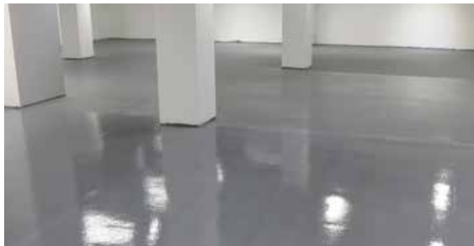
topcoat application with 322 C FLOOR Duo
