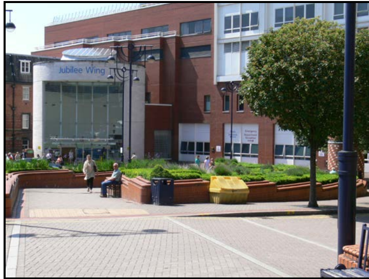
Figure 1, Leeds General Infirmary
