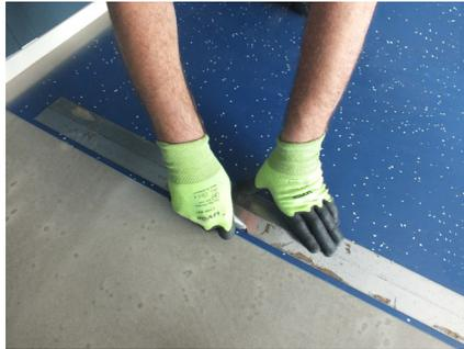
Trace the line of the trimmed edge onto the subfloor with a pencil. This line acts as a guide line.
