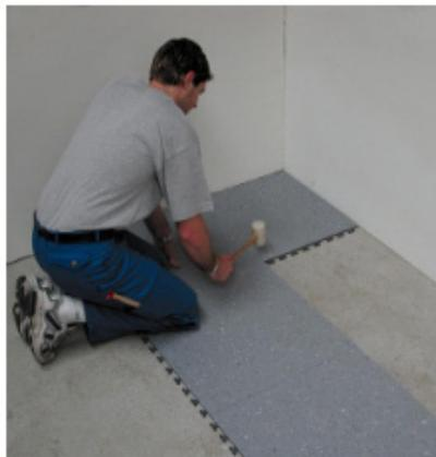
A rubber mallet can be used for engaging the connection system.
