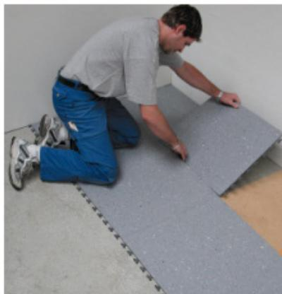
When inserting the border tiles, the second row must be slightly lifted.
