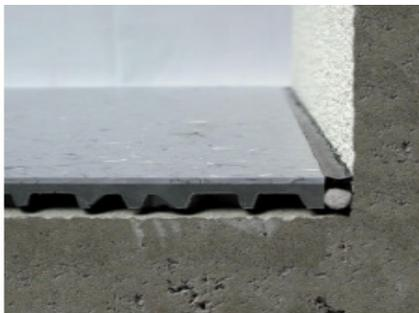
Correct! Lateral adhesion of PUR sealing compound. A foam cord is inserted first for optimum result.
