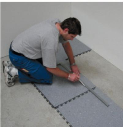
Mark out the cutting edge and cut with circular saw or jigsaw.
