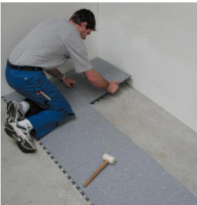
Once the second row is complete, the first row is measured and fitted.
