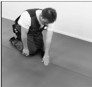
Cut the Forbo foam to fit the floor area and place it on the floor aluminum side upwards. Join the seams with the overlapping aluminum tape.
