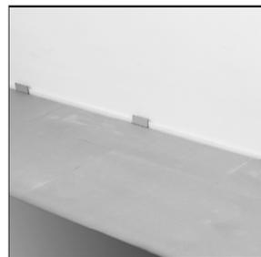
Place a row of full-size 3 mm panels (coloured adhesive uppermost) staggered against the first row of the cut panels - ideally in a brick design as shown above.
