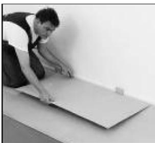
Place a row of full-size 4 mm panels (clear adhesive downwards) overlapping the second row of the 3 mm panels halfway. Install the remaining panels, covering the whole area in this manner.
