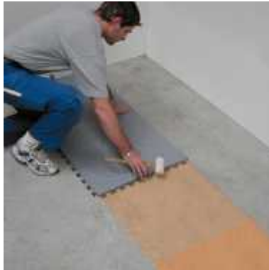
It is important that the second row is installed exactly along the chalk line.
