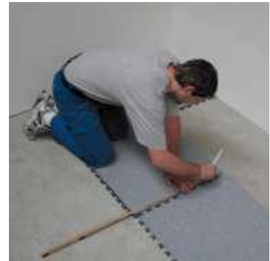
When measuring the border tiles, sufficient distance from the wall (gap) shall be allowed.
