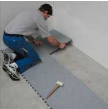
Once the second row is complete, the first row is measured and fitted.
