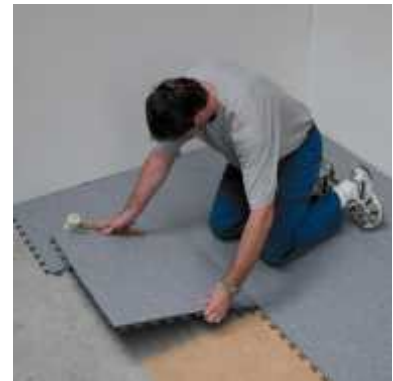
Once the first two rows are complete, the entire area can be gradually laid.
