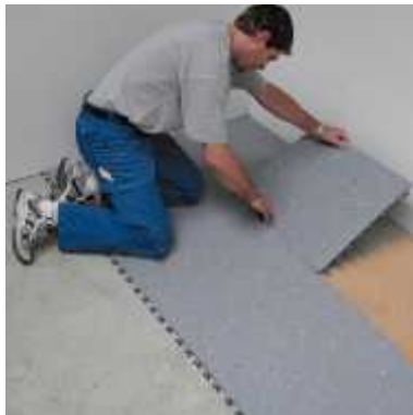
When inserting the border tiles, the second row must be slightly lifted.
