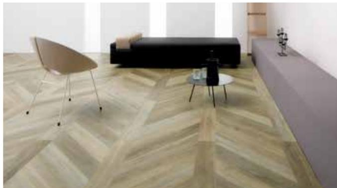
**Note:** As with any geometric design, irregularities or undulations in the subfloor can result in the bond of tiles or planks drifting during installation. This is particularly important with the installation of Hungarian point planks if the points of the planks are to meet consistently and particular attention should be given to the preparation of the subfloor to ensure that the highest level of subfloor regularity is achieved i.e. within SR1 surface regularity standard
