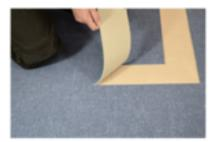
Apply a fresh layer of acrylic adhesive. Lay the *Flotex border* into the adhesive after the appropriate waiting time specified by the adhesive manufacturer and using a rubbing board press the border firmly into the adhesive (see below).
