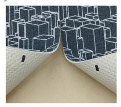
Dry lay the pieces, butting the factory edges for seaming. Make sure that the seam edges come together with a net fit with no fullness or gaps and check the pattern match.
