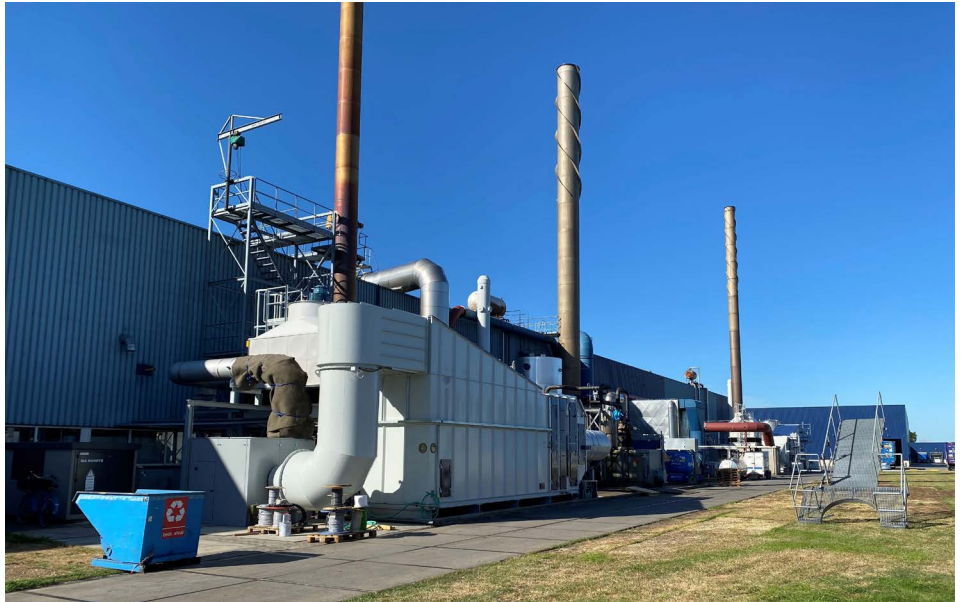
Coevorden, new filter technology installation.
