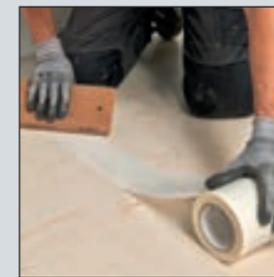
**2** Mark out the position of the Modul'up sheets on the subfloor. Apply the Modul'up adhesive tape, non-slip side down, along the marked joints and along door thresholds.
