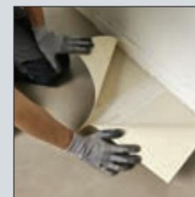
**3** The tape must be positioned so that both sheets cover the tape. Place the floor covering in the room, so that it covers the entire surface and laps up slightly along the walls (+10 cm).
