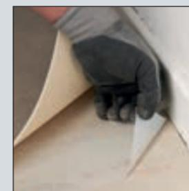
**4** Trim around the edges, but avoid cutting in too tightly (leave a gap of 1mm). Skirting can be fitted for a more aesthetic finish.
