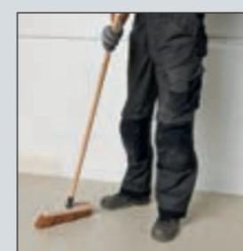
**1** Brush or vacuum the subfloor. In case of a new substrate, apply a primer.
