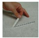
4. While still warm, remove excessive parts of the stripe with the crescent shape knife and/or sharp scraper and then allow the repair to cool down completely.
