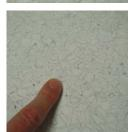
6. Complete by restoring the original surface smoothness of the repaired and grinded spot by dry polishing with a blue pad first and then with a red one. You can skip this passage if a restorative maintenance is to follow.
