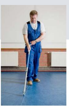
The upright cutter allows quick, controlled and easy cutting. Using standard hook blades, it is easily attached to the telescopic shaft.
