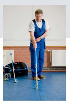
Trimming a welded seam has never been so quick and easy! First, trim roughly by using the standard welding slide .The final trimming can be performed when the weld cable has sufficiently cooled. A specially developed blade guarantees optimum quality for the welded surface.
