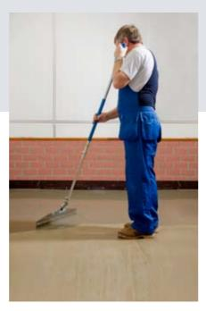
The screed-gauging tool is suitable for the application of all types of cement based levelling screeds. The trowel kit is adjustable, so that the correct working position can be obtained. The unique swivel joint helps to achieve perfect results. The screed blade is interchangeable.
