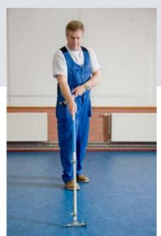
Scribing, using the trolley scriber is not only easier but also timesaving. When the scriber is accurately set to the correct angle, it is easy to scribe in a quick, controlled and ergonomic way.
