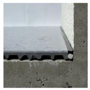
Correct! Lateral adhesion of PUR sealing compound. A foam cord is inserted first for optimum result.
