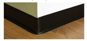
4. Backing Rod and coloured PUR caulking for discrete finish (NAB) example
