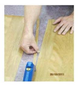
The narrow selvedge should be trimmed to within 2 to 3mm of the print line or along the print line of the plank depending on the installer's preference for the location of the welded seam.
