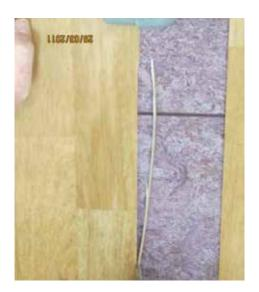
After trimming, the plank that contains the welded seam this may be slightly narrower than the main body. This will be lost in the overall design of the finished floor.
