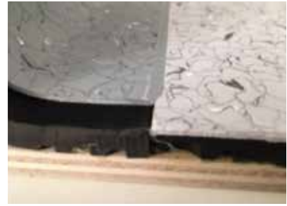
Welded cove former and tile
