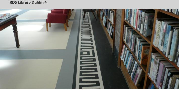
Following Detailed surveys of the existing patterns and selection of materials, including sample matching of the cream, white and blue colours of the original flooring, Forbo Marmoleum was specified and successfully used in the project. The large main flooring tiles were factory cut prior to delivery. The replacement border comprised the same Forbo material with the intricate pattern replicated in colour and design by cutting with an aquajet, also in factory conditions.
