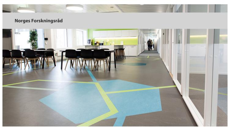
Norges Forskningsråd is an office for research scientists located in Oslo, Norway. The floor design is composed from various Marmoleum colors and the lines and figures were cut on place by the installers.
