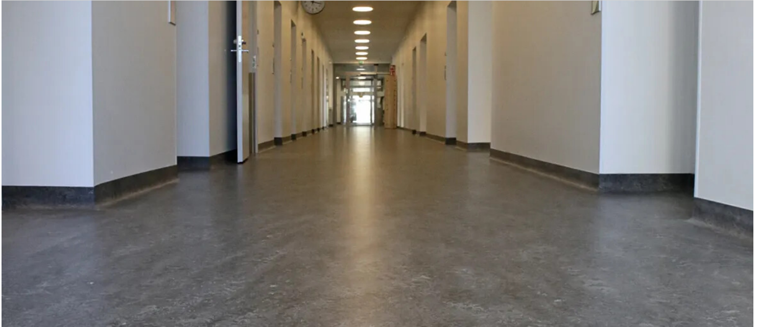
Hospital in Oulu, where installed 7000 m2 Marmoleum Real and 280 m2 Marmoleum Dual.
