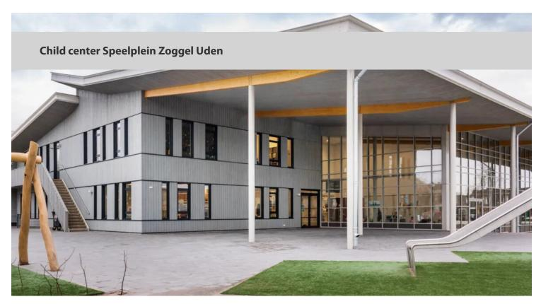
This child center is currently the most sustainable primary school in the Netherlands and is heated by means of an ice cellar. This is done according to the reverse refrigerator principle. The heat that is released during the cooling of the ice is used to heat the school building. Not only by using smart building techniques and installations such as rainwater collection for the toilets, but also by using many natural materials such as our CO2-neutral Marmoleum.
